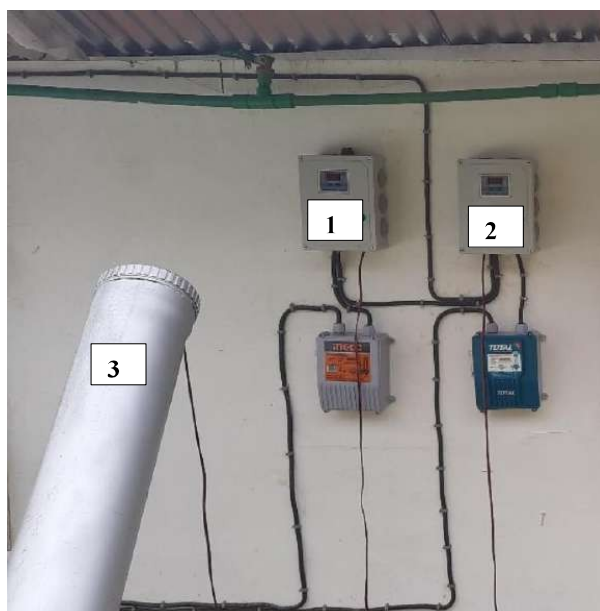
Photo 8. Dashboard for measuring the temperatures of the digester and digestate.
